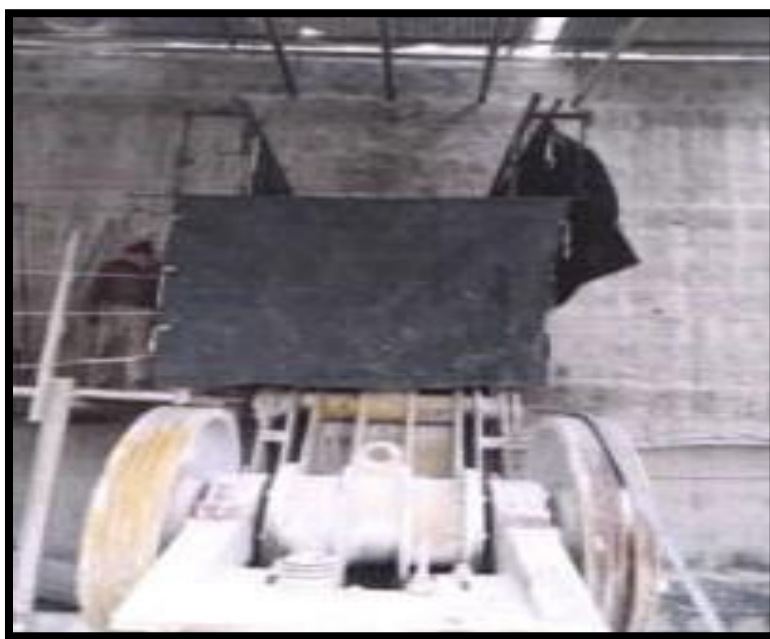
Figure-1: Covering of Primary/Jaw crusher
